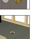
Mix modifed thinset as per manufacturer's instructions. Apply thinset to the subfloor starting at the back of the shower area, troweling towards the front. Ensure the trowel lines are pointing to the front or curb of your shower pan. This will ensure there will be no voids in the installation. DO NOT cross channel trowel lines or air can
