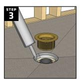
Apply a continuous ¼" bead of HYDRO-BLOK Joint Sealant around the top edge of the first notch inside the shower drain profile ensuring that the bead is consistent and full. Drop the solid brass drain body into the joint sealant and seat it firmly.
