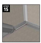
Apply a continuous 1/2" bead of joint sealant into the corner seams of the pan where it meets the wallboard. Use the corner putty knife to smooth out the sealant so that there is at least 1" of sealant on either side of the seams.
